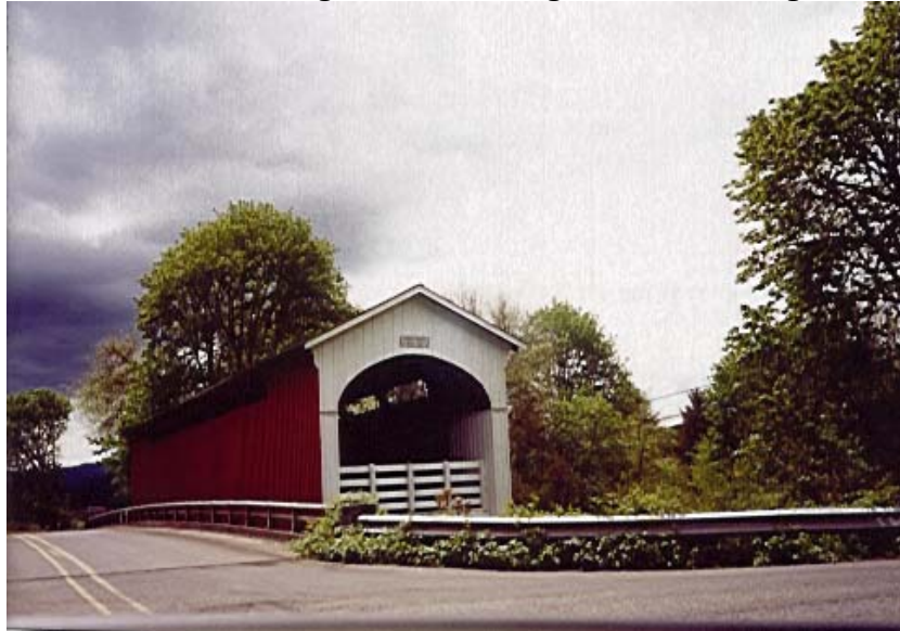
Figure 82 The Currin Covered Bridge Near Cottage Grove Dating From 1925
