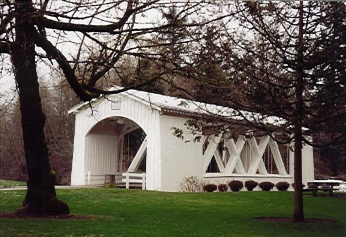
Figure 17 Stayton's Jordan Bridge, Built in 1998
